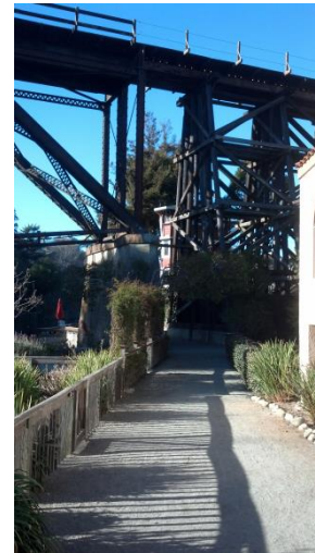
Looking north, before the trestle
