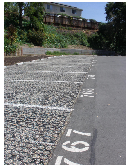
Permeable surface parking spaces have gravel held in place by a mat of plastic cells
